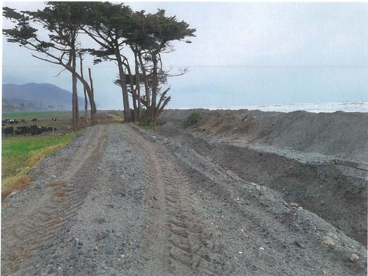
Primary and sacrificial bunds rebuilt.
