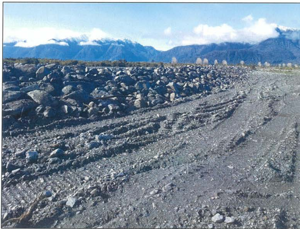
Completed extension of stopbank with rubble riprap
