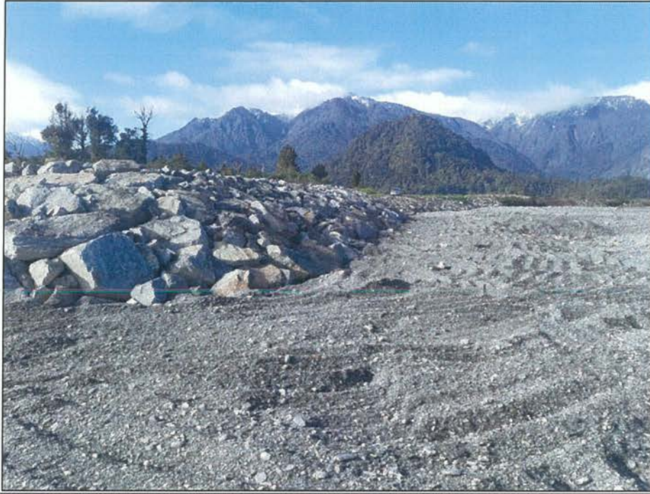
Structure #10 rock riprap repair
